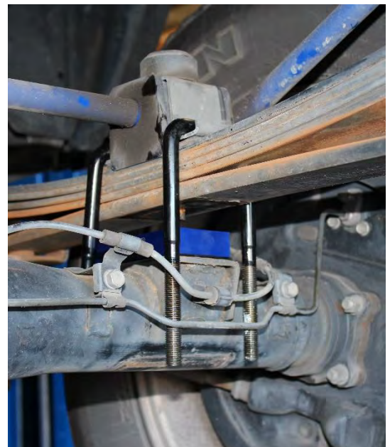
Picture 3: Installation of Raising Block
